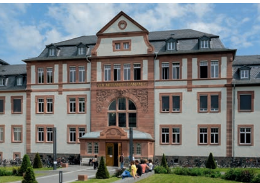
Fig. 12 Auditorium building: Following renovation and extension work, the medical lecture hall building now unites previously separate teaching sites and offers ideal studies and teaching infrastructure together with the surrounding University Hospital buildings.
